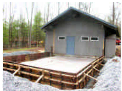
Construction site showing concrete forms.
